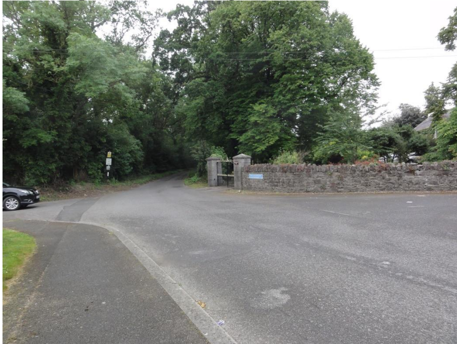
Leixlip Gate entrance together with mature trees.
